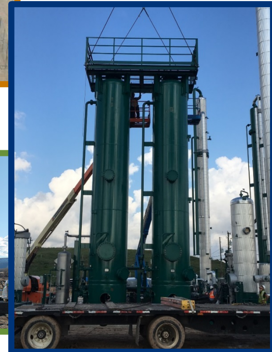
Seabreeze Landfill Angleton, TX
